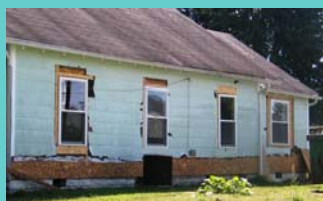
Home in Hurricane that received new windows from Storehouse WV
